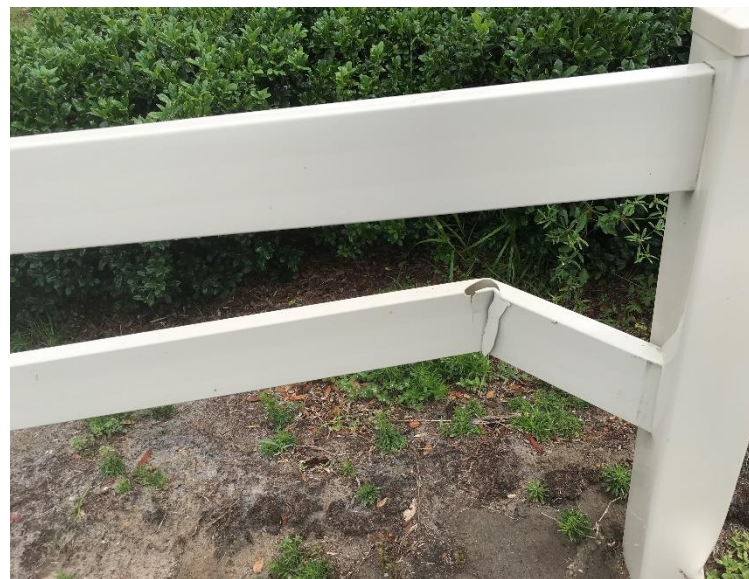
Repaired broken fence
