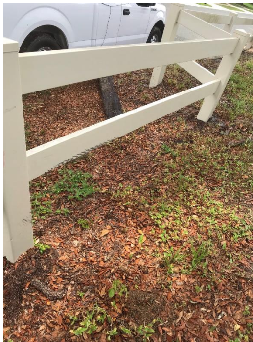
Pressure washed fence
